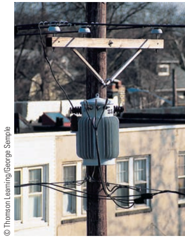
This transformer is smaller than the one in the opening photograph of this chapter. In addition, it is a step-down transformer. It drops the voltage from 4 000 V to 240 V for delivery to a group of residences.
